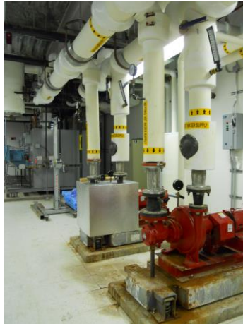
Figure 8: Hydronic mechanical-hot water pumps
